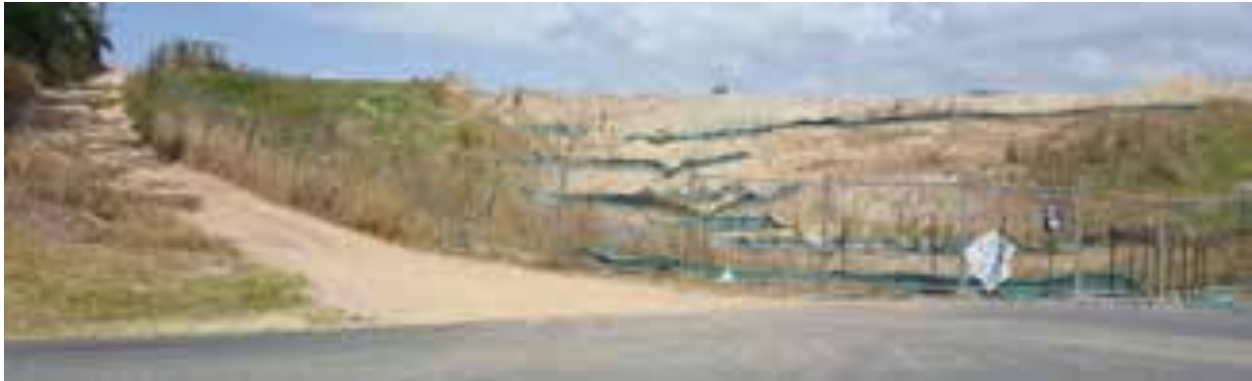
Stalled development at Woolgoolga Heights
