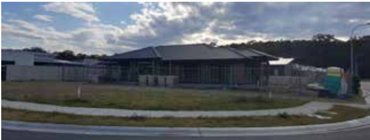
Detached housing construction at North Sandy Beach
